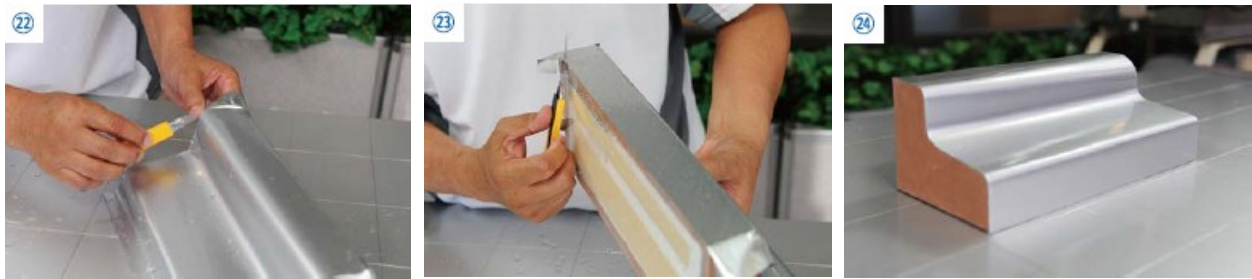
Trim the edges of the film with a sharp tool while the film is still wet. Finish the film edge with a spatula.
